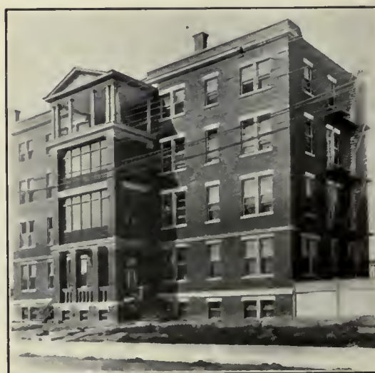
St. Justine Hospital, St. Denis Street. Joseph Sawyer, Architect.
